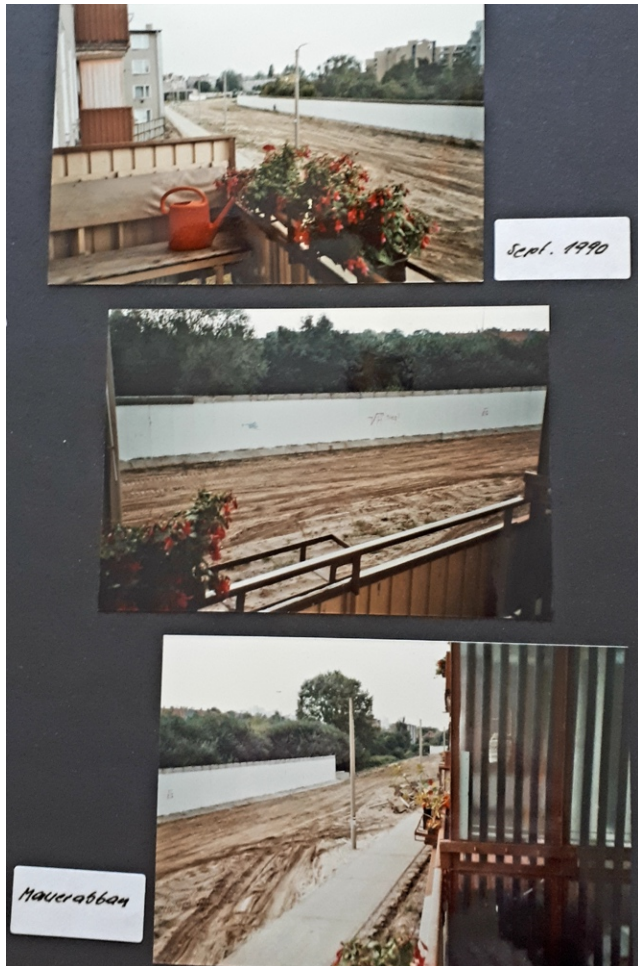
Dismantling of the Berlin Wall. Berlin-Baumschulenweg, September 1990. (Photograph by Hanno Schmikale) 2
