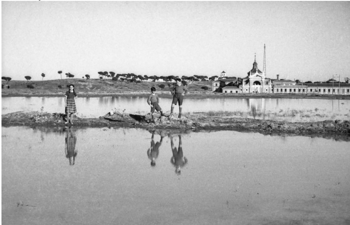
The Convento de las Madres Reparadoras, which housed Military Hospital No. 6, is in the background of this photo from 1949. Today, the area is densely built-up. 76 Image: Manuel Urech.
